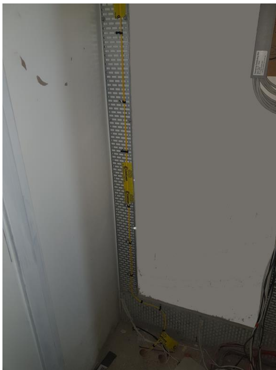
Figure 5 - Examples of Vertical Telecommunications Pathways
